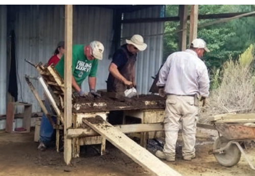
The team from Robinhood Road, led by Karla Hackworth, worked hard to produce adobe block, which will be used throughout the year at the construction site.
