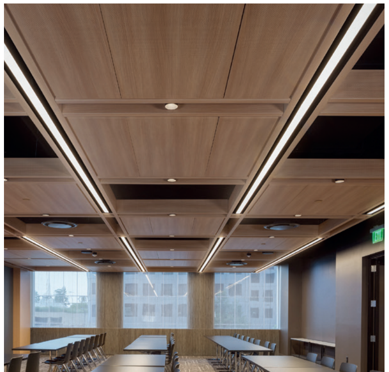
PROJECT: 400 Atlantic PRODUCT: AERO:Form™ Parallel Open Cell with acoustic panels
